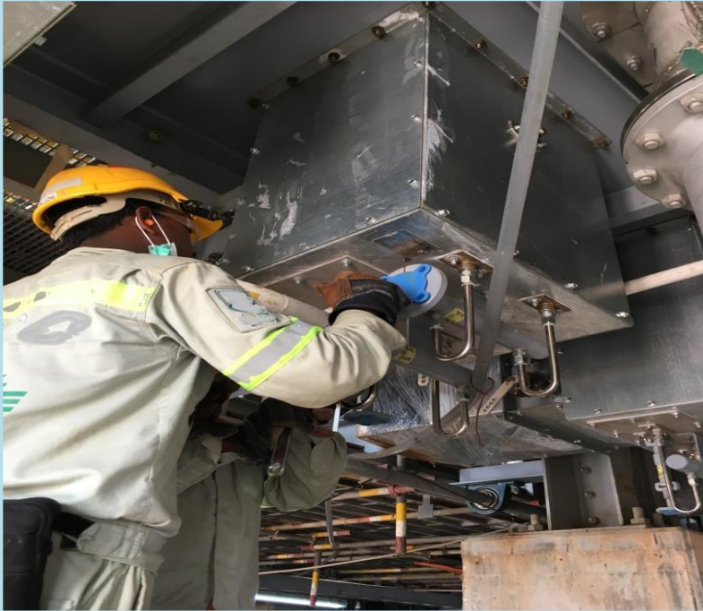
➤ Furnace Burner Equipment Installation
