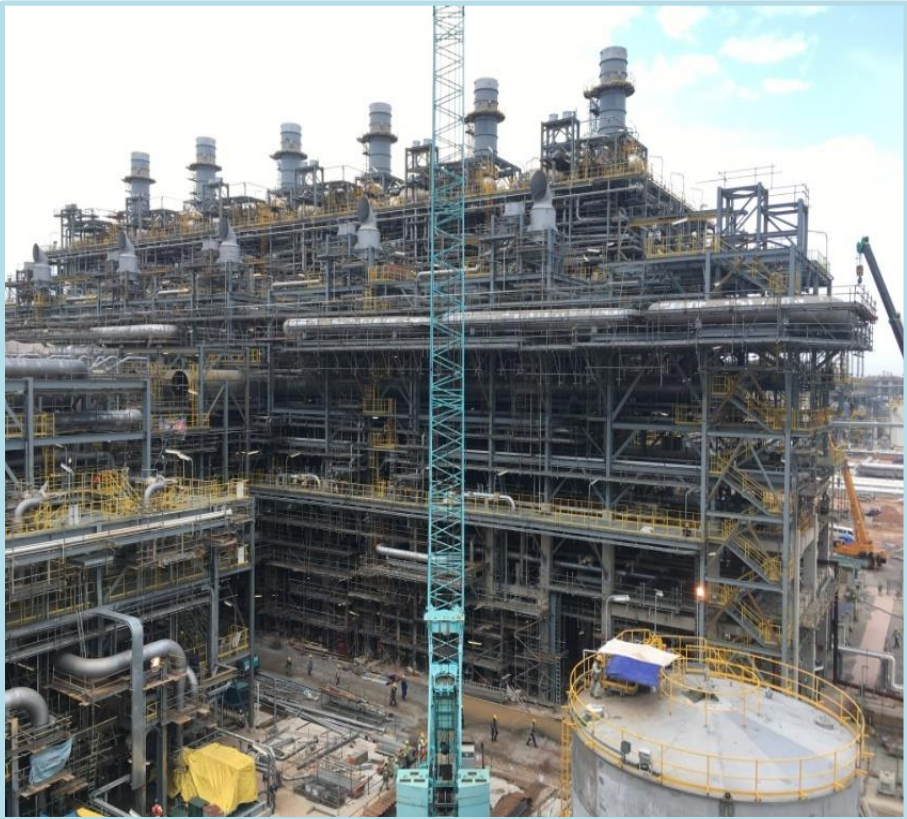
➤ Furnace end view together with Pipe rack ➤ Pipe rack pipe spool installation by Fong Leong
