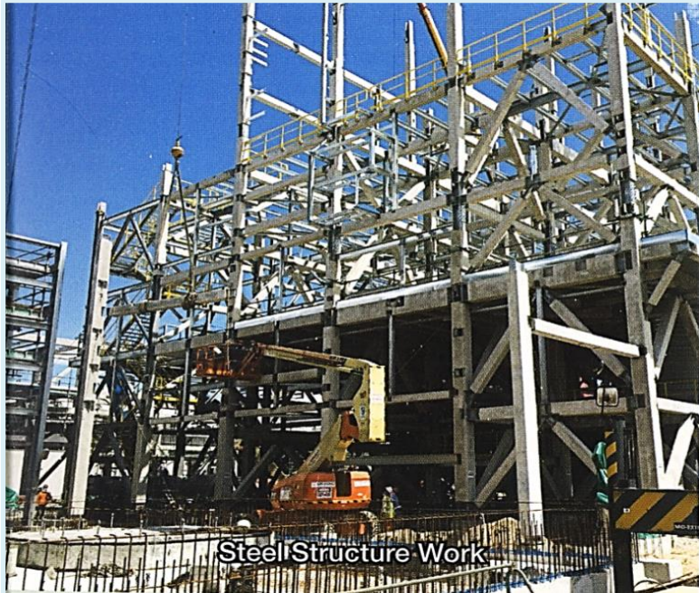
Steel Structure Work
