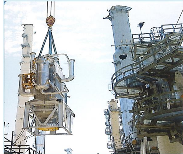
Installation of Heavy Equipment Work
